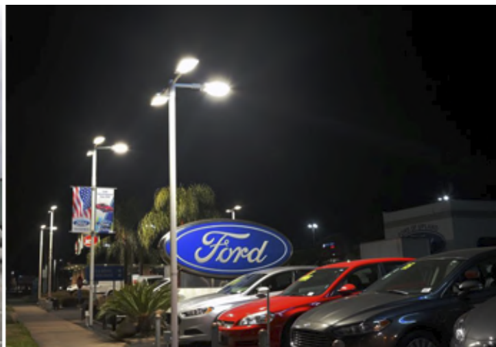
Long Beach Port — LED Shoebox light replacement
